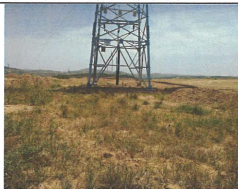
杆塔周围生态恢复
